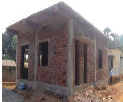
Construction of School Building at Govindpauram Village
