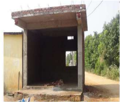
Construction of School Building at Govindpauram Village
