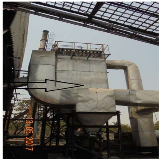
Photographs of Existing Boilers Stack connected to Bag Filters
